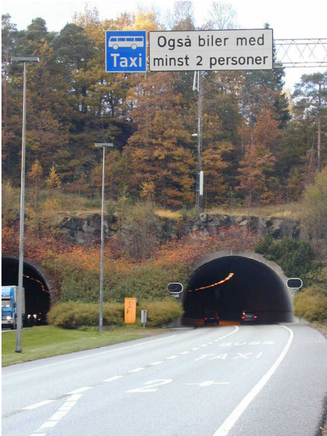
Figure 2: Signs and marking from the start of the HOV-lane in Kristiansand.
